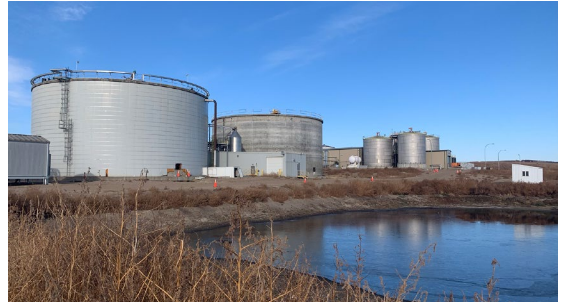
The Two Hills RNG facility will capture enough RNG from organic waste to power 2,500 homes.
