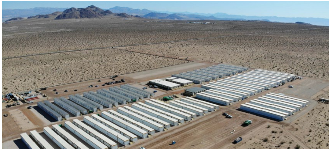
ATCO provided workforce housing and lodging services at Naval Air Weapons Station, China Lake, near Ridgecrest, California.
